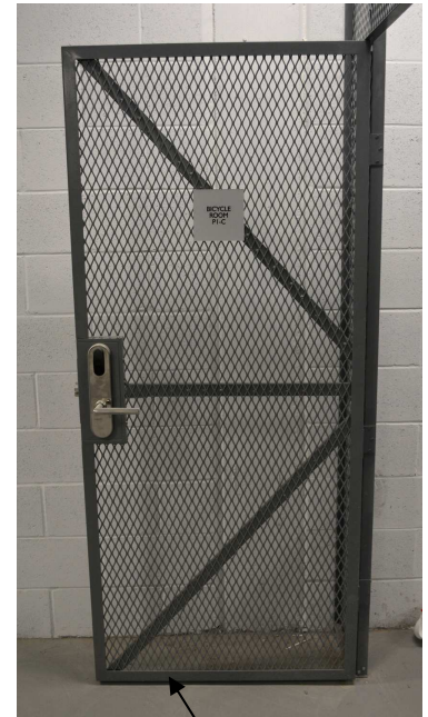
Custom expanded sheet metal door
