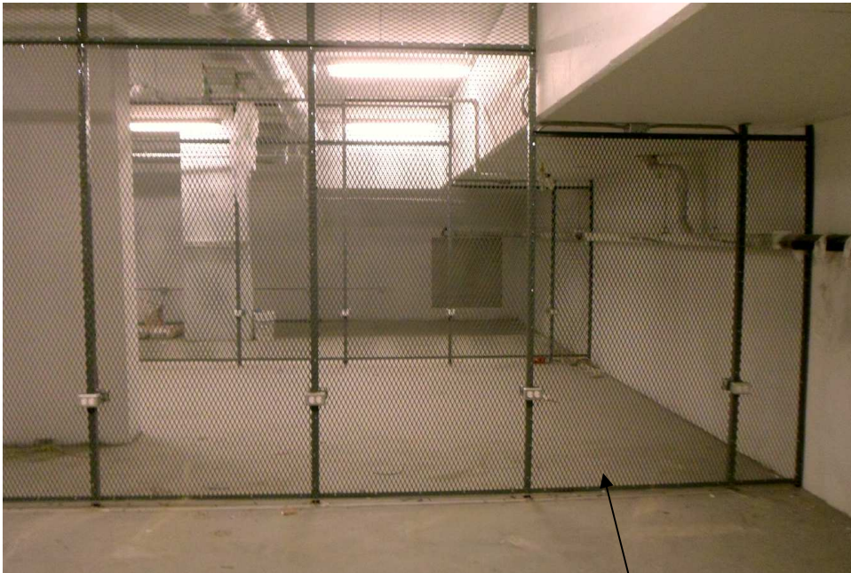
Floor to ceiling partition installation
